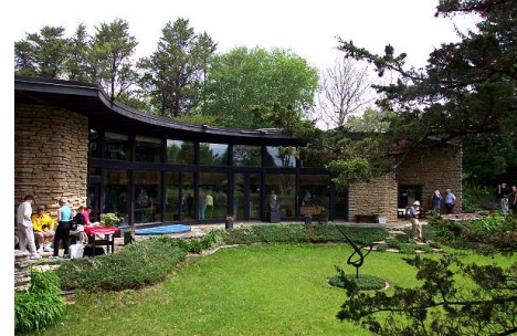
Figure 1: The Jacobs II House. The glass facade faces south to maximize passive solar heating. Image from www.dgunning.org .
